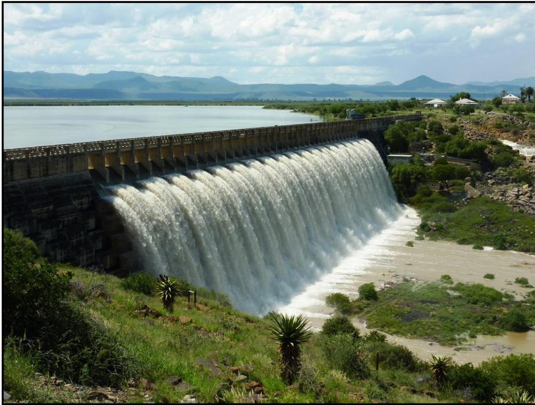
Nqweba Dam overflowing on 11/02/2011
